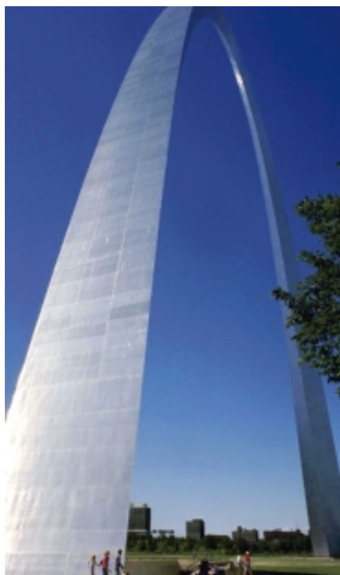
Reflecting on the future: convergence of technologies will have a big impact on the building automation industry.
